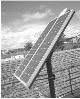
Figure 1: Modules installed on the structure support.
