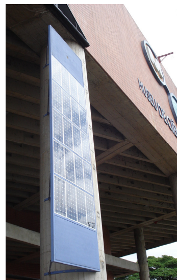
Fig. 1. PV system installed in the façade of the Science and Technology Museum of the PUCRS, Brazil.
