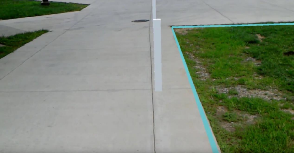
Figure 41 – Two virtual columns added to a known feature (junction in the concrete ground), and a virtual line that shows the border of the pathway.
